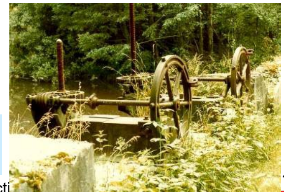
Condition of hydromechanical equipment
